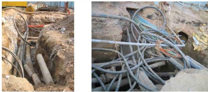
Figure 1. Typical utilities were found in one of the metro projects in Delhi [8]
