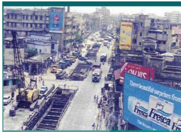
Figure 3. Cut and cover construction through Chittaranjan Avenue (Som, 2017).
