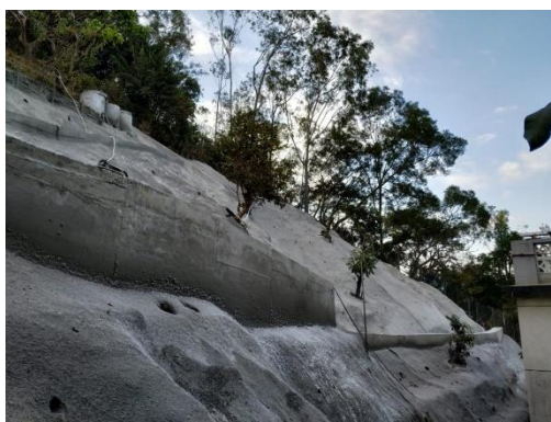
Plate 3-29: Slope surface with covered with fibre-reinforced shotcrete.
