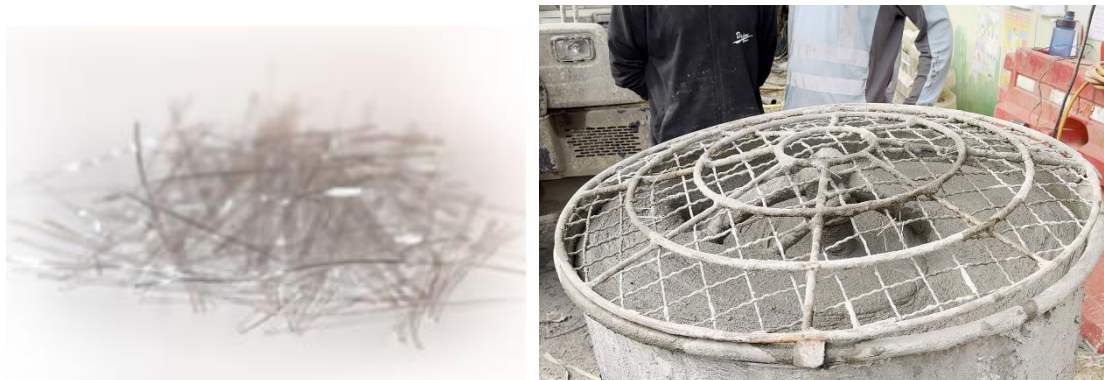
Plates 3-24 & 3-25: Mixing of fibre-reinforced shotcrete for shotcreting works
