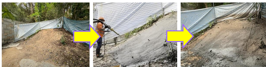
Plates 3-26, 3-27 & 3-28: Typical working procedures of shotcreting works using fibre-reinforced shotcrete. Original slope surface (left); application of shotcrete (middle); shotcreted slope surface (right).
