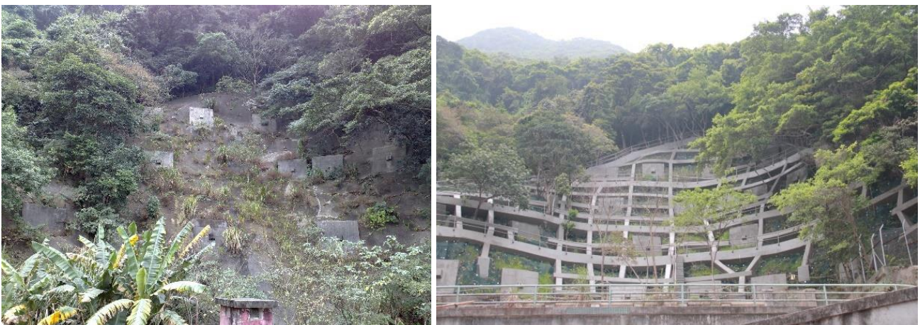
Plates 3-1 & 3-2: Subject government cut slope: before upgrading works with heads of ground anchor exposed on slope surface (left); upgrading works with grid beams exposed on slope surface (right)
