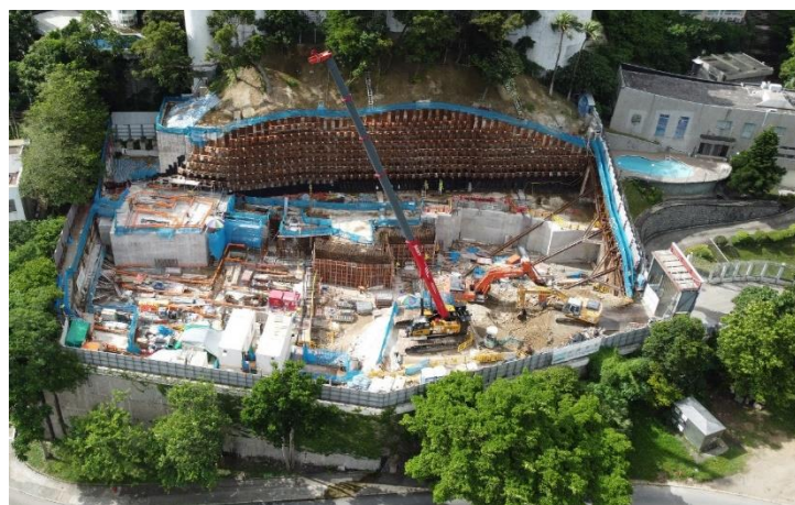
Plate 4-3: Photo Showing Completed Anchored Soldier Pile Wall (with Tie Back) in Residential Development at Deep Water Bay
