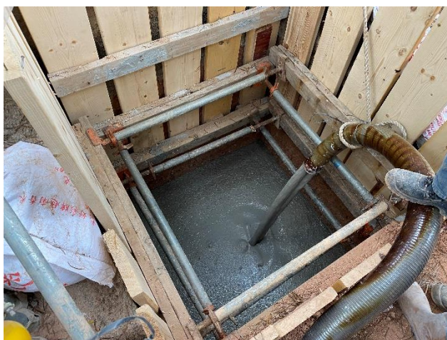
Plate 3-17: Backfilling of a pit by self-compacting material during site trial
