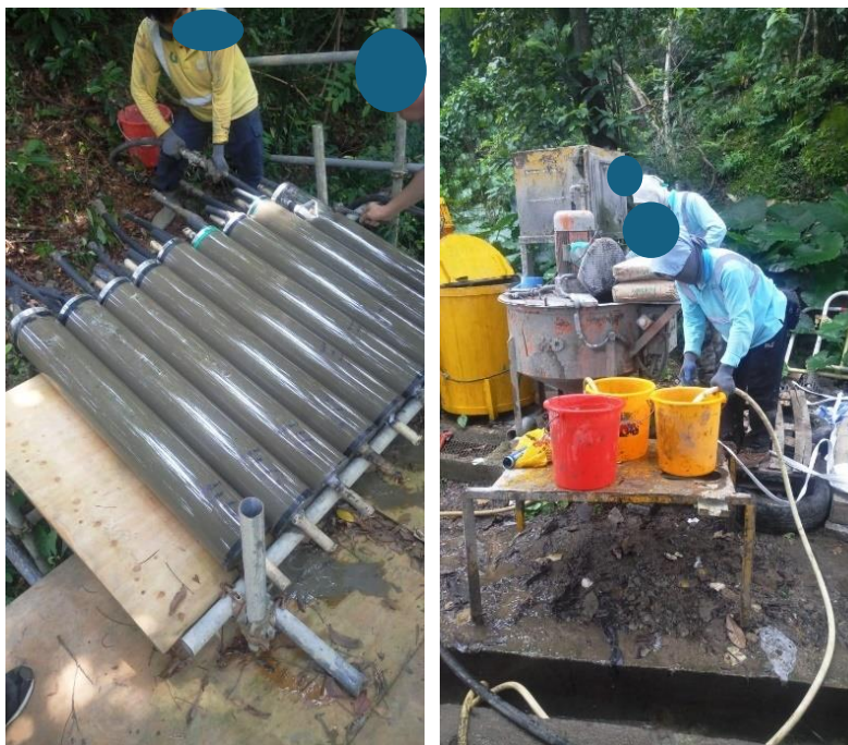
Plates 3-15 & 3-16: Filled moulds for simulated grouting exercise (left), mixing of ECC grout during site trial (right).
