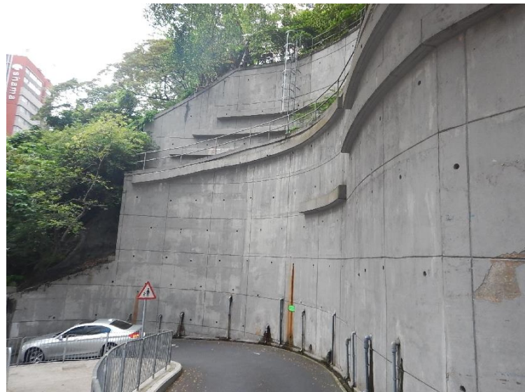
Plate 3-3: General view of the retaining wall after completion of upgrading works.
