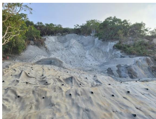
Plate 3-23 : Extent of emergency slope surfacing works under Concrete Canvas
