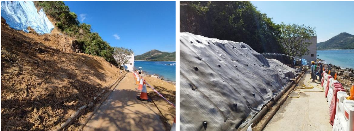
Plates 3-21 & 3-22: General view of the slope surface before (Left) and after (Right) emergency slope surfacing works using Concrete Canvas
