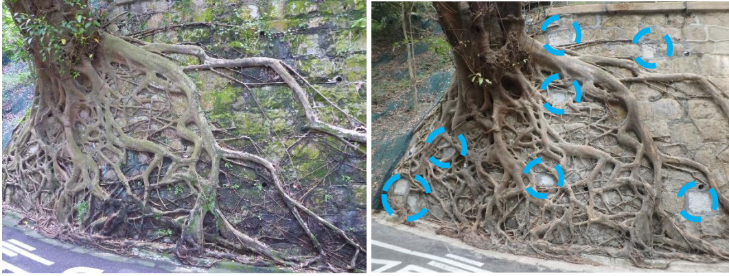
Plates 3-4 & 3-5: Root portion of the stone wall tree: before installation of soil nails (left); after completion of soil nailing works. Locations are soil nail heads are circled in blue. (right)
