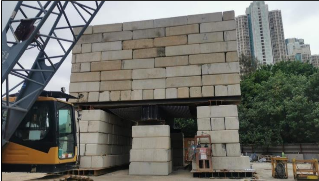
Plate 2: Kentledge set up for load test
