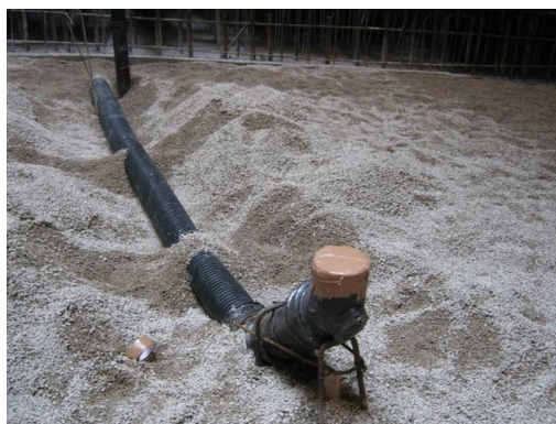
Plate 1: Rodding eye connected to horizontal perforated pipe inside drainage layer
