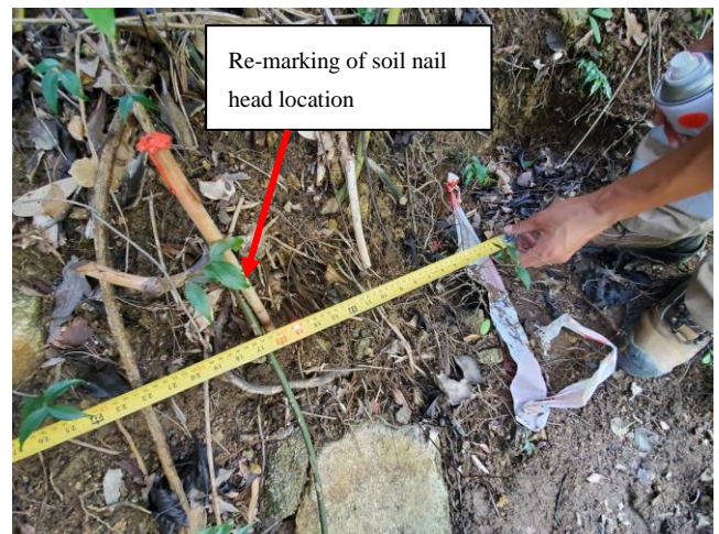
Plate 16: Re-marking of soil nail head locations at Row BG
