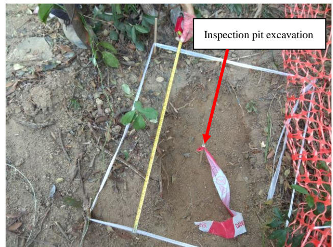
Plate 14: Inspection pit excavation for Row BF Soil Nails
