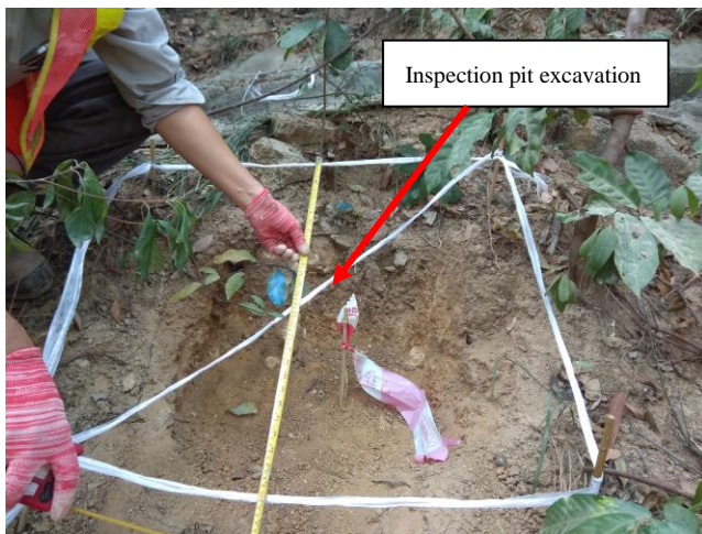
Plate 13: Inspection pit excavation for Row BG Soil Nails
