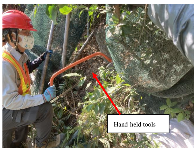
Plate 11: Only hand-held tools were allowed for selective trimming. Plant identification and extent of trimming was confirmed by the Ecologist before trimming.
