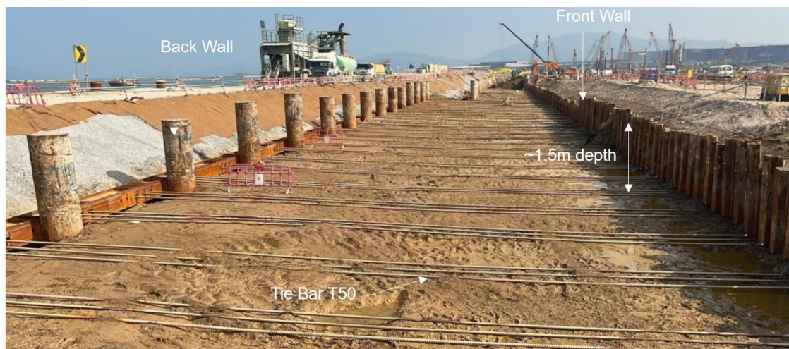
Plate 2: Shallow excavation for tie installation
