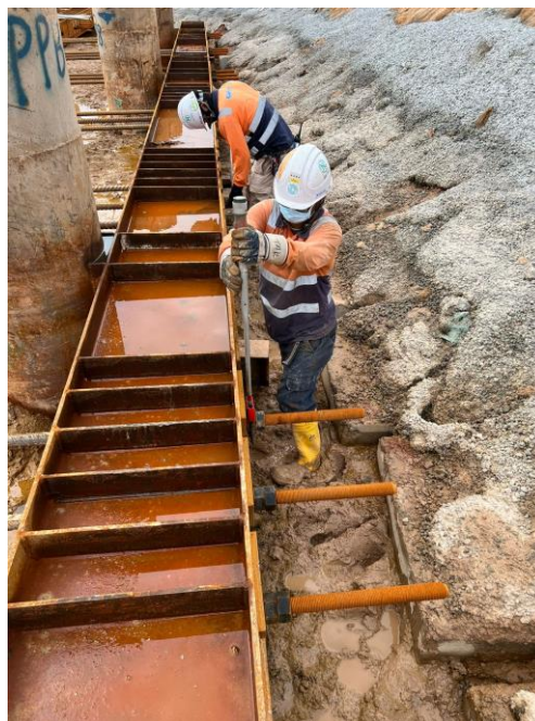
Plate 4: Tie connection installation
