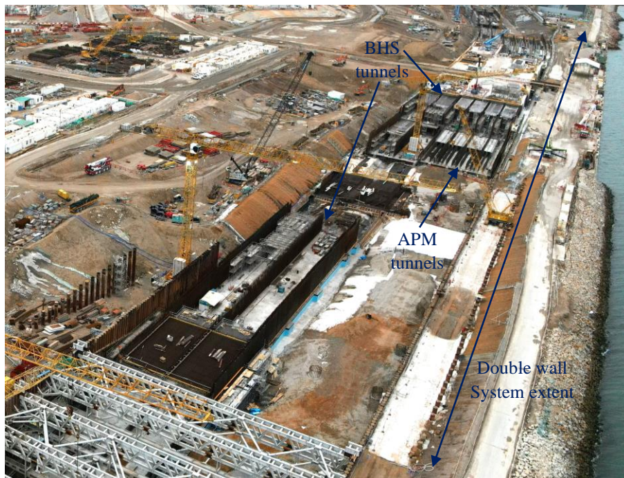
Plate 8: Construction of tunnel structure in spacious area
