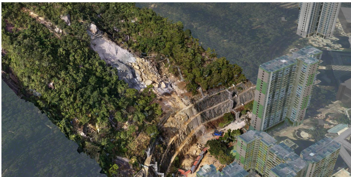
Figure 6: Condition of the landslide site at Yiu Hing Road in February 2024
