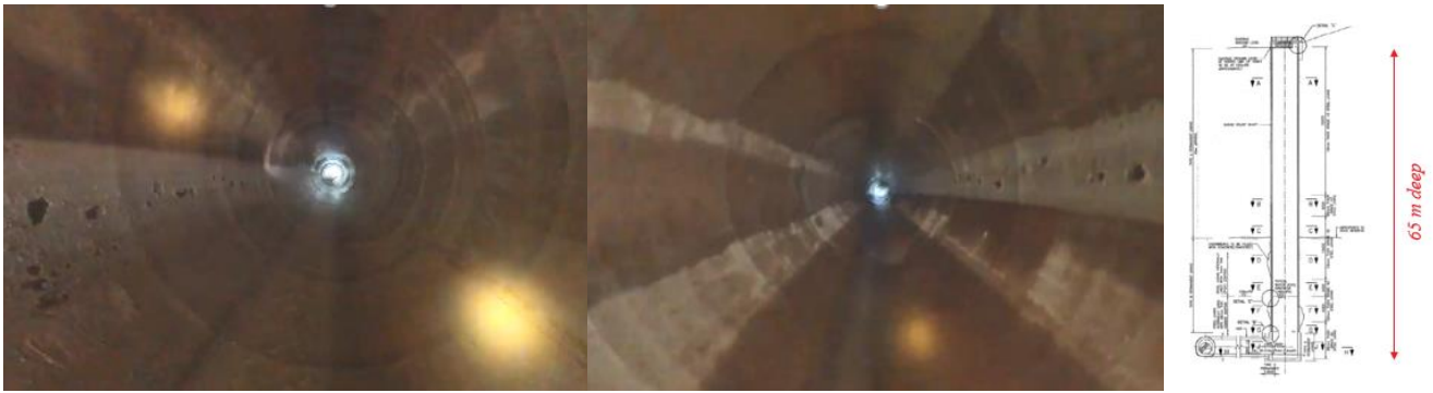
Figure 12: Inspection of Inaccessible Shafts
