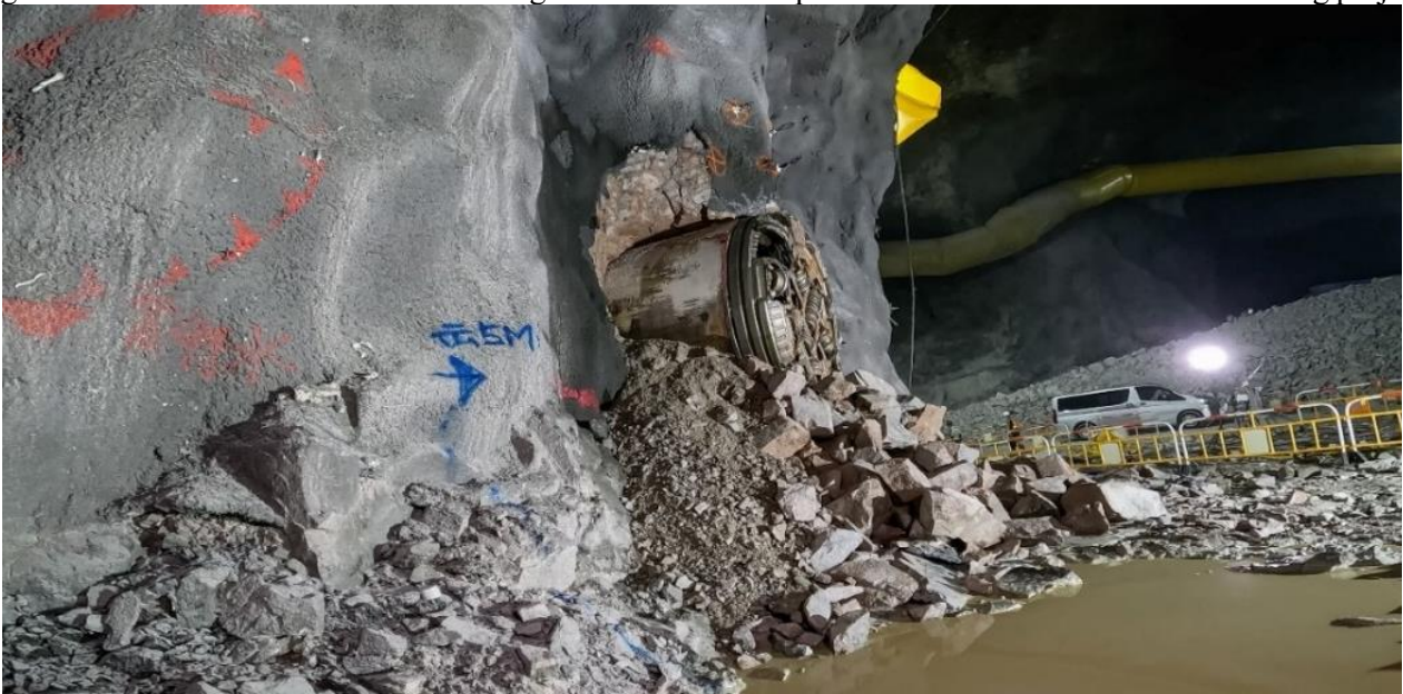
Photo 6 – Successful completion of 1 st effluent pipe
