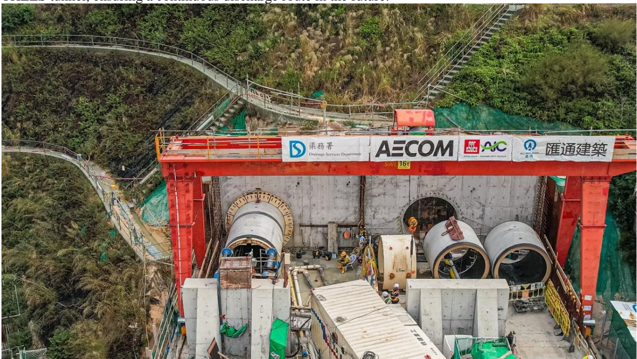
Photo 1 – General view of jacking thrust structure and lifting gantry
