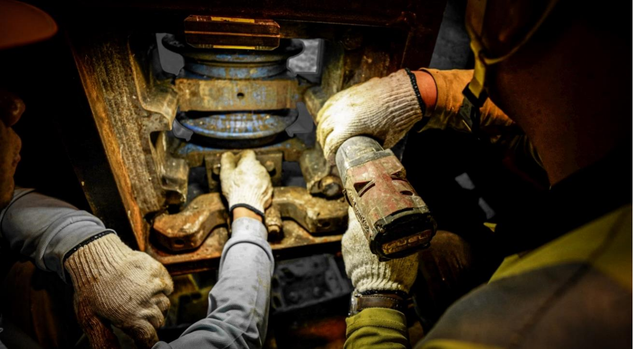
Photo 5 – Replacement of cutter disc
