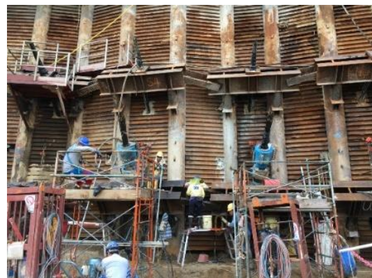
Plate 8: Jacking of Anchors in Progress
