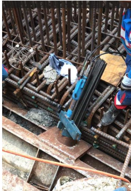
Plate 9: Removal of strands in Progress
