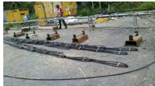
Plate 3: Fabricated Anchor Units
