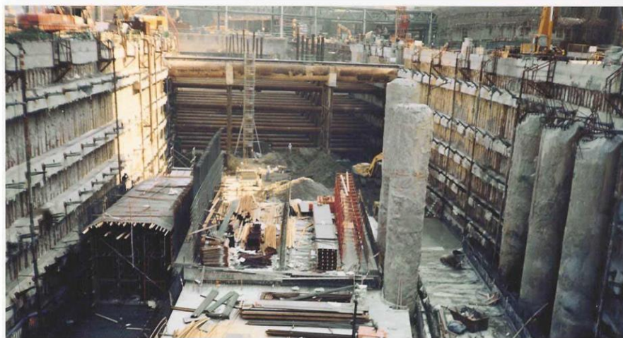
Photograph 3. 200-tonne working capacity multiple anchors at Central Station in Hong Kong.
