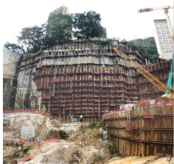
Plate 6: General View of Completed ELS Works
