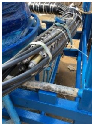
Plate 7: Anchor Body before inserting into Drillhole
