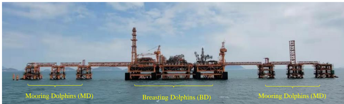
Figure 1: Photograph of the completed foundations of HKOLNGT (Lee et al, 2022)
