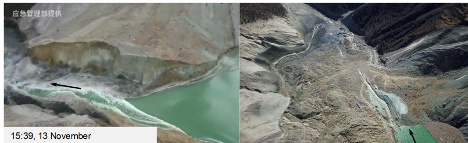
Figure 2. The Jinsha River landslide dam breaching in November 2018.
