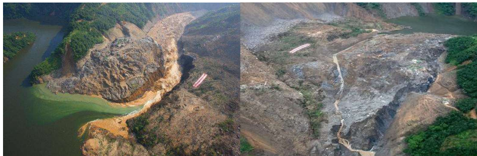
Figure 3. The Tangjiashan landslide dam breaching in June 2008.
