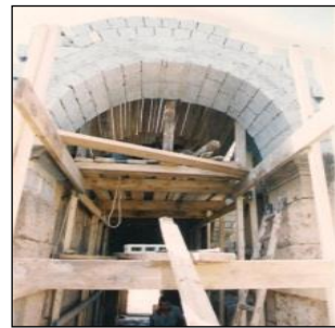
Figure 12: Using the limestone bricks to roof the western entrance of the theatre [10].
