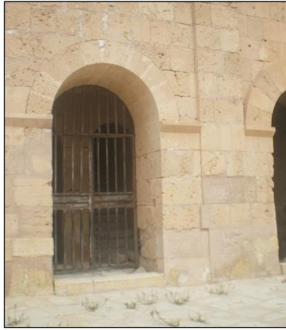
Figure 5: Treatment of arcs using materials of the same original building material [5].
