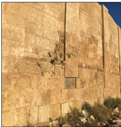
Figure 15: Using the cement blocks in the restoration of outer wall (Authors, 2018)
