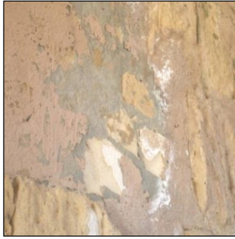
Figure 8: Using concrete in the floors and surfaces,(Authors,2012)
