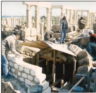
Figure 10: Using the cement block in the theater[10].
