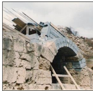
Figure 11: Using concrete and reinforcement steel in the roof of the eastern entrance of the theatre[10].
