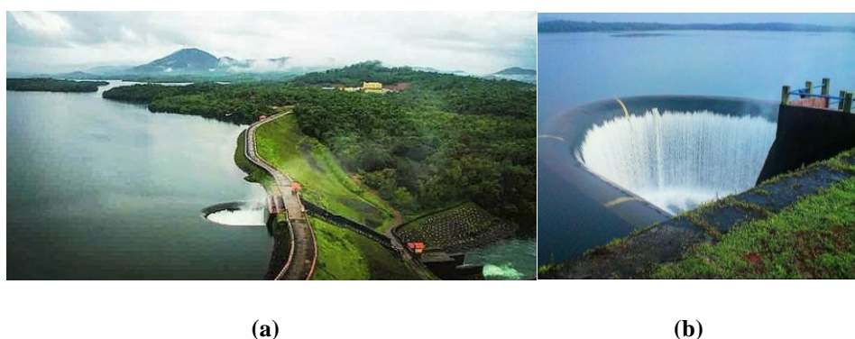
Figure 1 (a) Salaulim Dam, Goa and (b) Duckbill Spillway at Salaulim Dam
