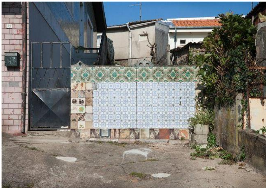
Figure 2: Wall with patchwork of tiles, 2023. Source: Authors.
