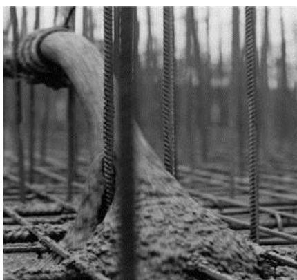
Figure 1: Pouring SCC between the reinforcement (Source: Rich et al., 2012)
