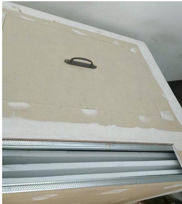
Figure 11: Scenario 4 - With EPS sheets -three layer in the centre of gypsum partition wall
