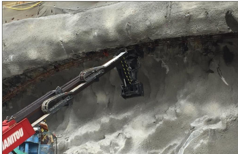
Figure 11: Installation of Lattice Girder Segment
