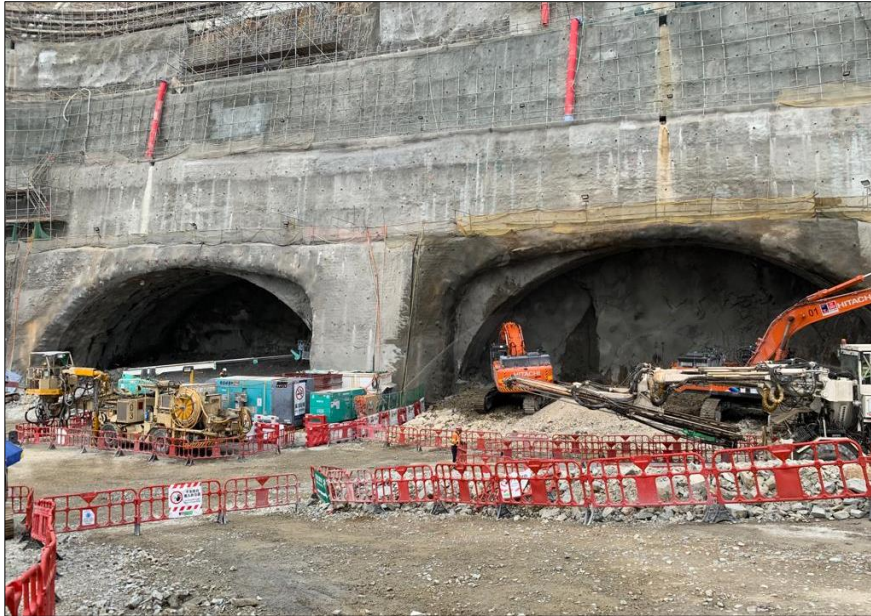
Figure 10: Top-heading Excavation by Mechanical Method
