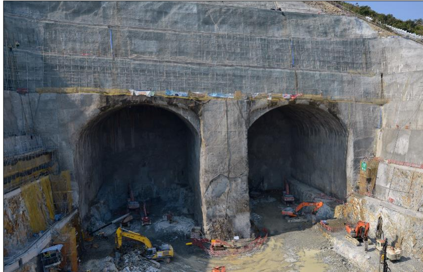
Figure 12: Cavern Bench Excavation and Portal Slope Site Formation Works
