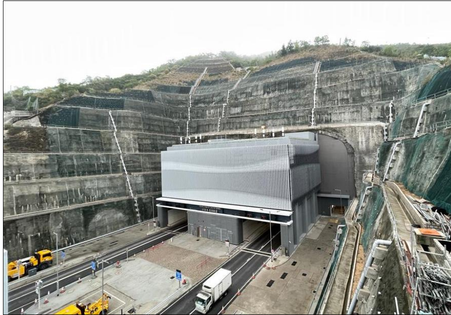
Figure 14: The completion of Semi-Cavern and EVB works
