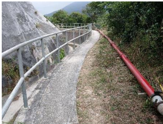
(c) Use of pipelines for transportation of SCM within the site (d) Placement of SCM by chutes
