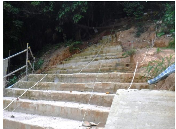
(b) Loose fill replaced by SCM
