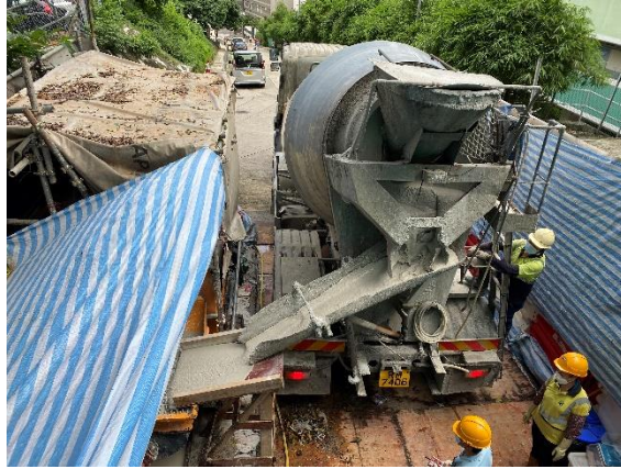
(a) Delivery of ready-mixed SCM by concrete truck (b) Discharge of ready-mixed SCM to concrete pump
