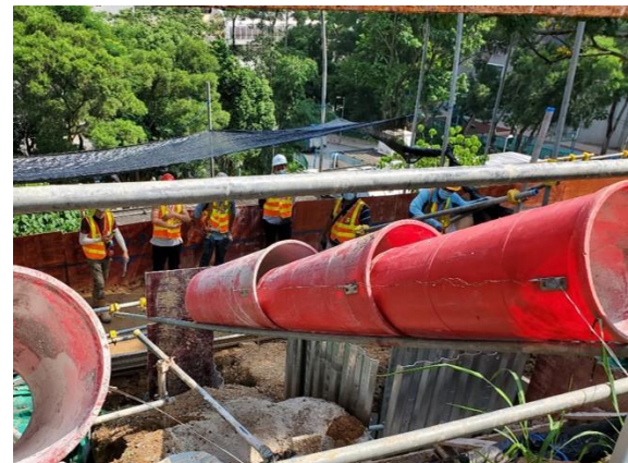
(c) Use of pipelines for transportation of SCM within the site (d) Placement of SCM by chutes
