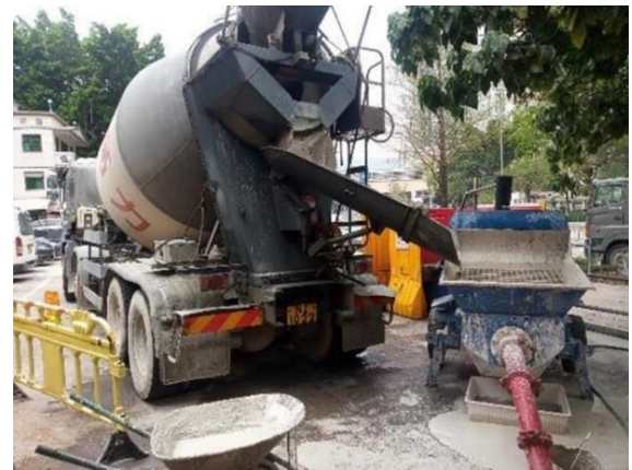
(a) Delivery of ready-mixed SCM by concrete truck (b) Discharge of ready-mixed SCM to concrete pump
