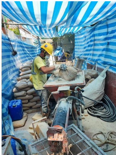
(a) Production of SCM using screw mixer on site (b) SCM discharged from the screw mixer
