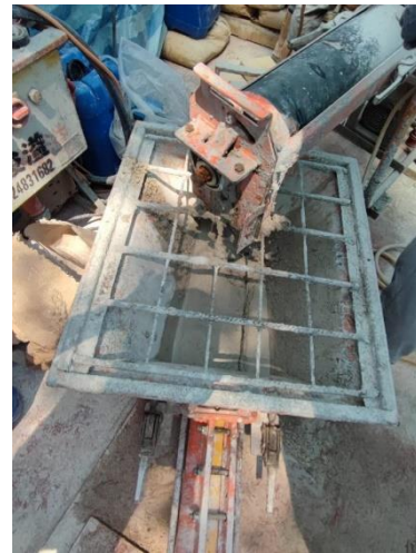
(a) Production of SCM using screw mixer on site (b) SCM discharged from the screw mixer
