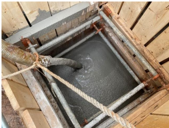
(a) Placement of SCM for fill replacement in a pit
