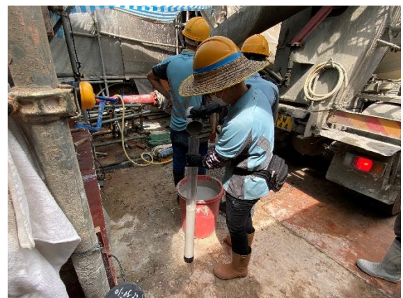
(b) Sampling and preparation of cylindrical sample for laboratory testing
