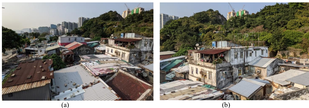
Figure 8: (a) Corrugated rooftop unsuitable for installation of GNSS rover station in CKL Village and (b) Rooftop occupied by antennas & prior consent from resident required for installing GNSS rover station
