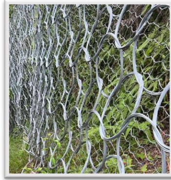
Figure 2: Photo of chain wire meshes and teel ring nets.
