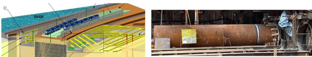
Figure 20: Installation of Canopy Tubes above Crown of Tunnel Boxes by micro TBM and pipe jacking
