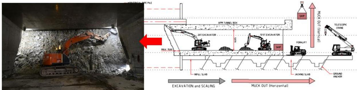
Figure 31: Excavation with the use of hydraulic excavator and breaker.
