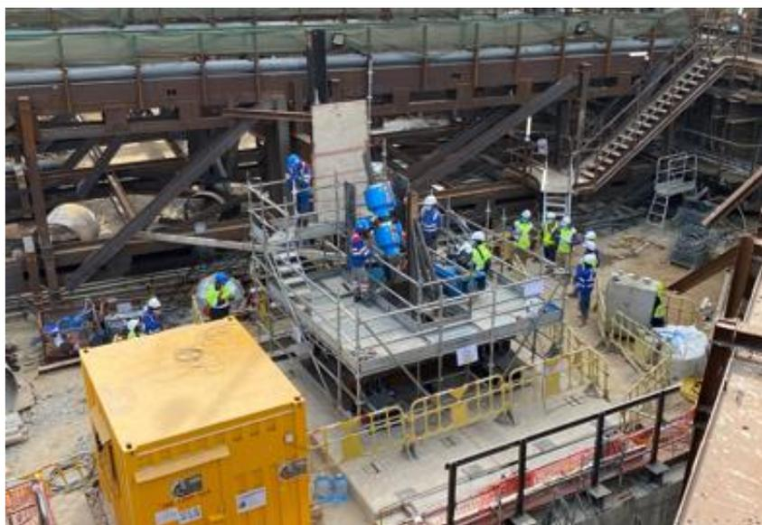
**Figure 26:** Ground Anchor Suitability Test Set Up
