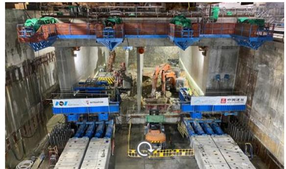
**Figure 22:** *Typical Arrangement of Jacked Boxes on Jacking Slab*
