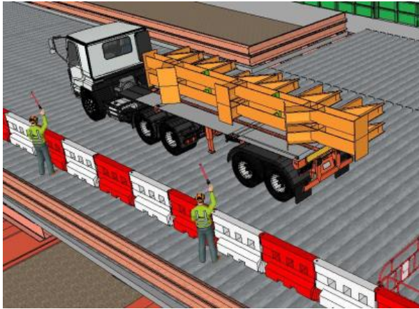
Figure 17: Digital Delivery of Modules to Site
