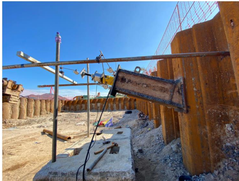
Figure 9: Set up of Pull out test on Site
