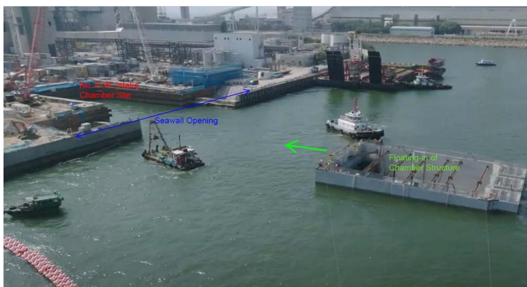
Figure 13: The ELS with seawall opening for receiving the floating caisson
