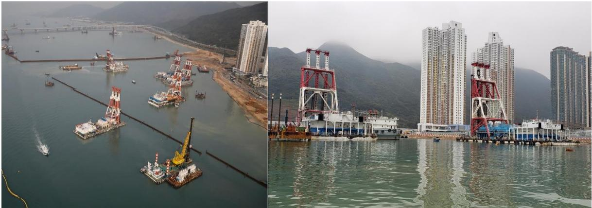
**Figure 10:** *Marine DCM barges on work close to residential area*
