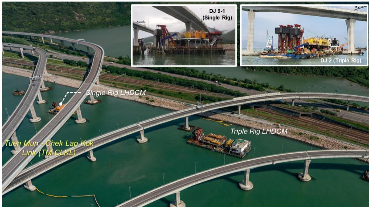
**Figure 18:** Two low headroom barges working under the TM-CLK Link
