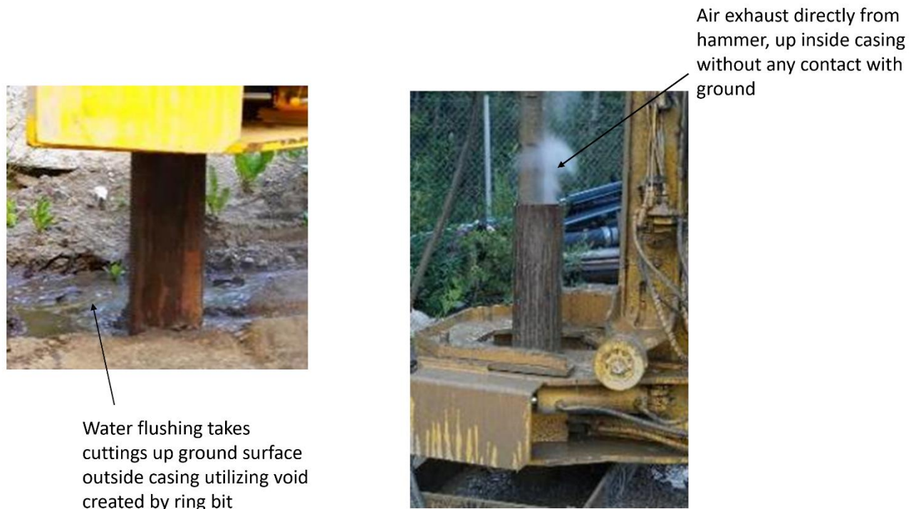
Figure 12: Flow paths of air and water during drilling using the ALF system
