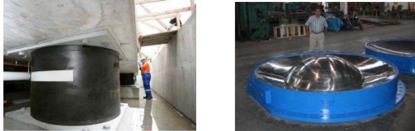
**Figure 1:** *Seismic isolation devices- (a) elastomeric bearing, (b) friction pendulum bearing.*
