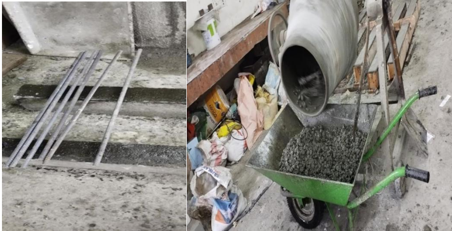
Figure 2: 16mm diameter reinforcing bar and concrete mix.
