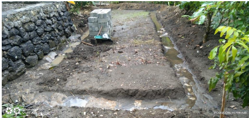
Figure 5: The process of making ponds for raising silkworms implemented at Klayar
