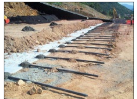
Geocomposite – Drainage layer Ma On Shan Development July 2021
