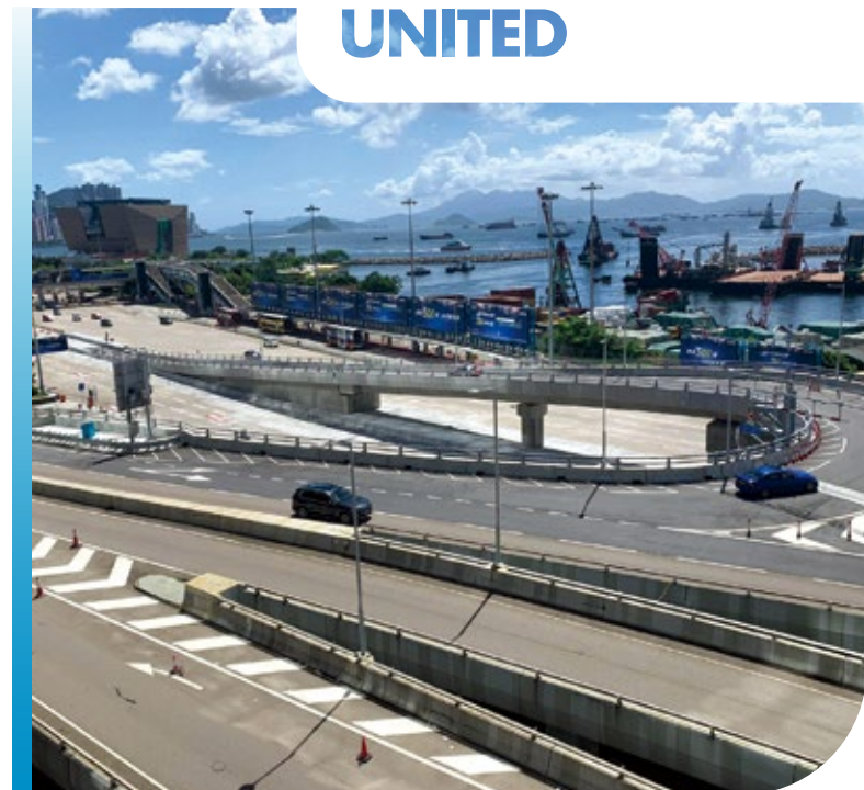
Road Improvement Works in West Kowloon Reclamation Development
