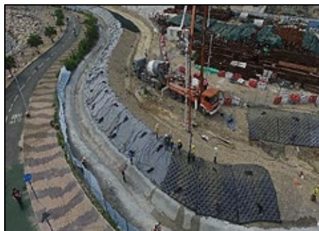
Concrete Mattress – Embankment for Coastal Protection TKO December 2017
