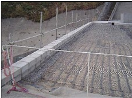
Geogrid - Reinforced Fill Wall NENT Landfill October 2005
