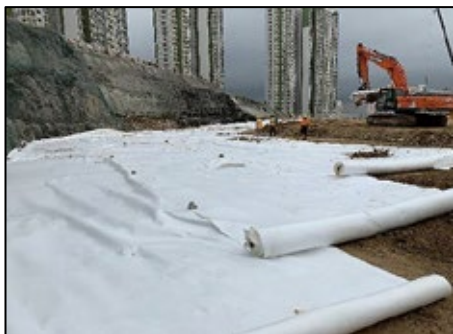
Geotextile – Formation Stability Anderson Road Development August 2017
