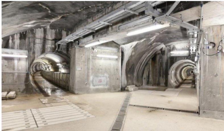
Figure 4: Intersection at Po Shan Road Drainage Tunnel with Permanent SFRS Lining
