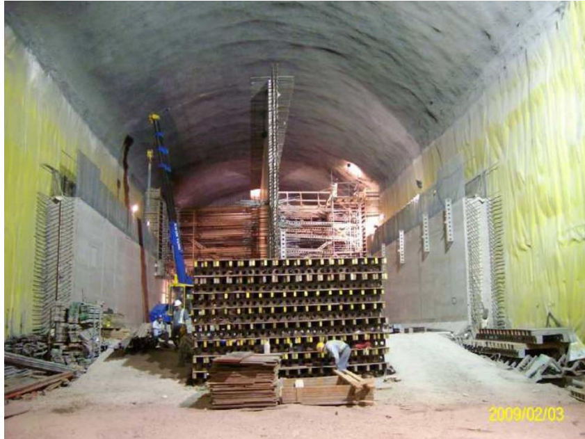
Figure 10: Construction of Western Salt Water Service Reservoirs at HKU
