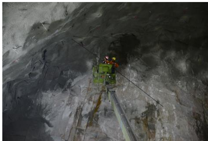
Figure 5: Rock Bolt Installation in Hard Rock
