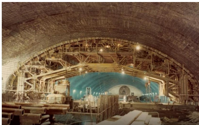
Figure 3: Steel Shutter for the Construction of MTR Tai Koo Station
