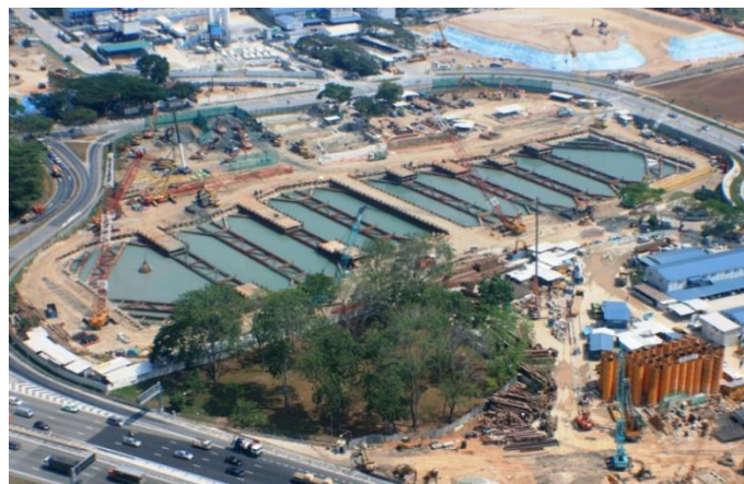
Plate 1: Mega-Truss concept as used for ELS works in Marina Bay, Singapore
