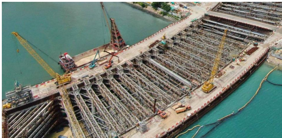
Plate 3: Completed view of skidding mega trusses at UWT Stage 1
