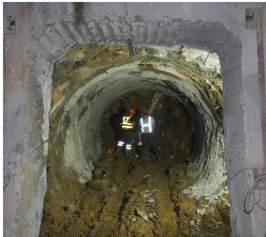
Plate 10: Cross Passage Excavation (View from Permanent Opening)
