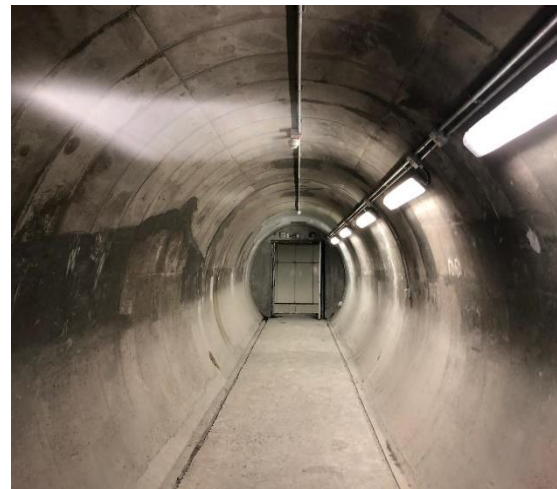
Plate 11: Cross Passage with Permanent Structural Lining
