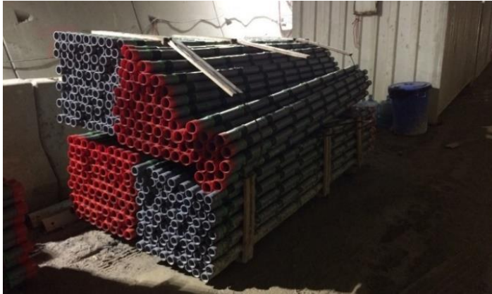
Plate 3: TAM Grouting Pipes
