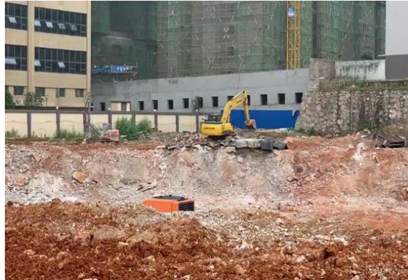
Figure 9: Basement excavation for building project using SC-CO 2
