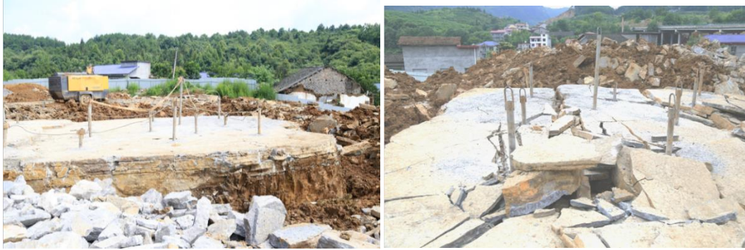
Figure 8: Site formation for highway project using SC-CO 2
