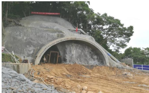
Figure 10: Tunnel portal excavation using SC-CO 2
