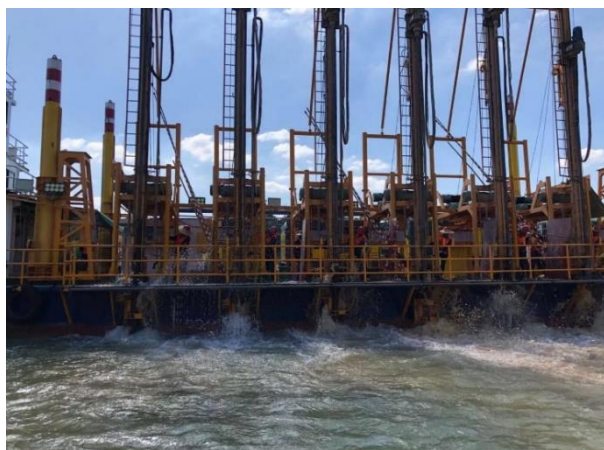
Figure 11: Underwater rock fracturing using SC-CO 2
