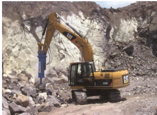
Figure 1: Hydraulic breaker mounted on backhoe
