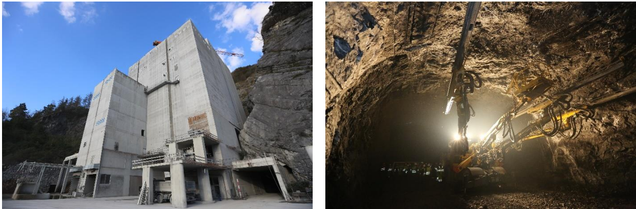
Plate 1: Schollberg Underground Quarry in Switzerland; (left) rock processing plant; (right) underground quarry excavation
