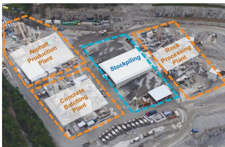
Figure 6: Typical ancillary facilities at surface portal site for underground quarrying
