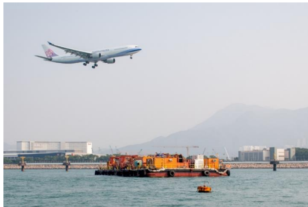
Figure 1: Marine CSM working in low headroom condition
