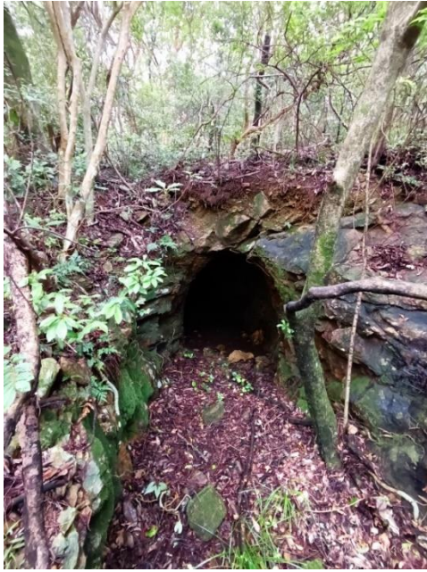
Plate 4: Adit identified by LiDAR integrated with API and field mapping.
