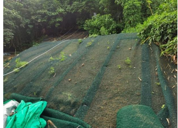
Figure 15: Slope works after placement of backfilling material (Lei Uk Tsuen)
