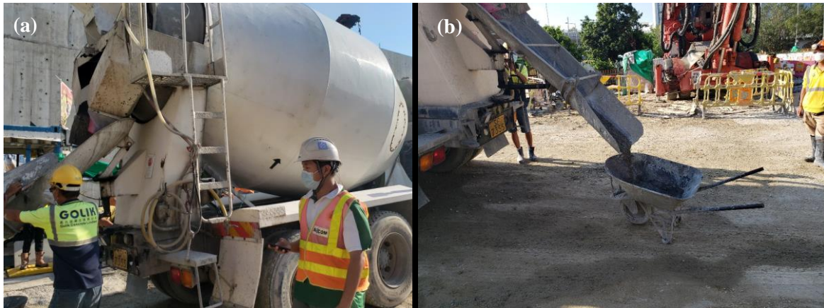
Figure 6: (a) The concrete truck arrived on-site, and (b) fresh VRSC was poured for testing
