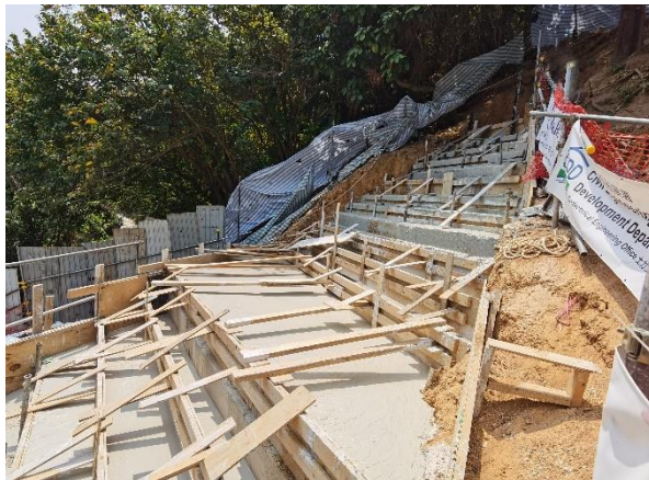
Figure 15: Slope works after placement of backfilling material (Lei Uk Tsuen)
