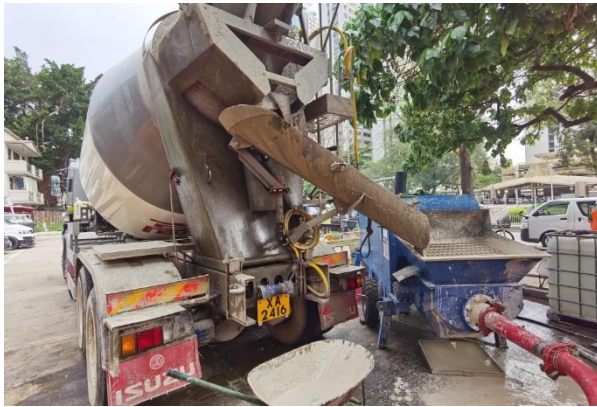
Figure 14: Pumping backfilling material from concrete truck to the pit (Lei Uk Tsuen)
