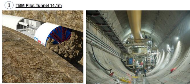
Figure 7: 315m long pilot EPB TBM fibre reinforced segmental lining tunnel
