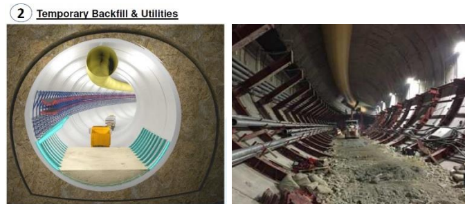
Figure 8: Installation of temporary steel gallery foundation, backfill and utilities
