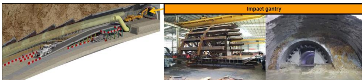
Figure 12: Special impact gantry preventing the fall of large blocks and reducing the impact load on the steel gallery
