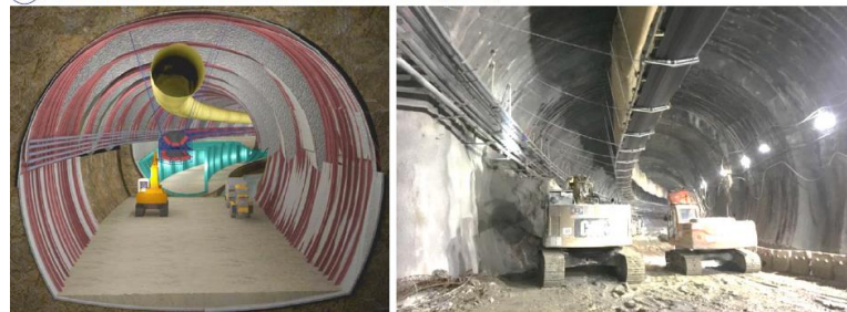
Figure 14: Left-hand side bench enlargement and completion of the steel gallery dismantling
