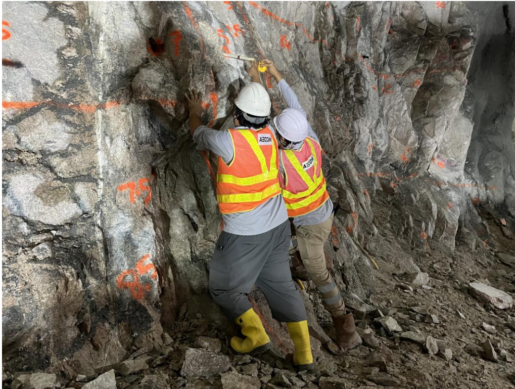
Photo 1: Depth Checking of As-built Blast Holes by Inserting a Ruler Manually
