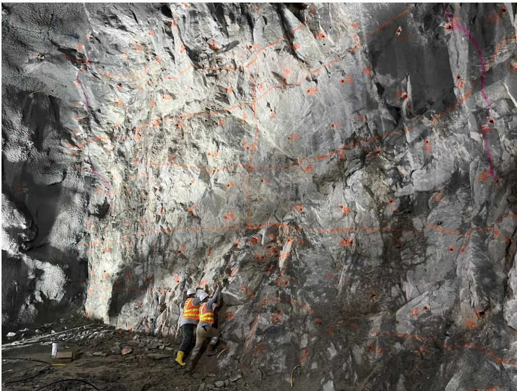
Photo 2: Depth Checking Covers Few As-built Blast Holes Only
