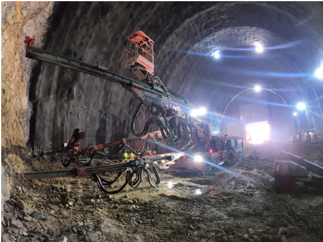
Photo 5: Jumbo Equipped with MWD Sensors
