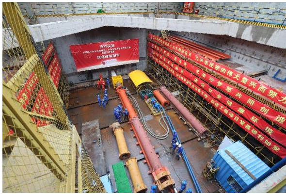
Figure 9A: Pipe curtain jacking in process
