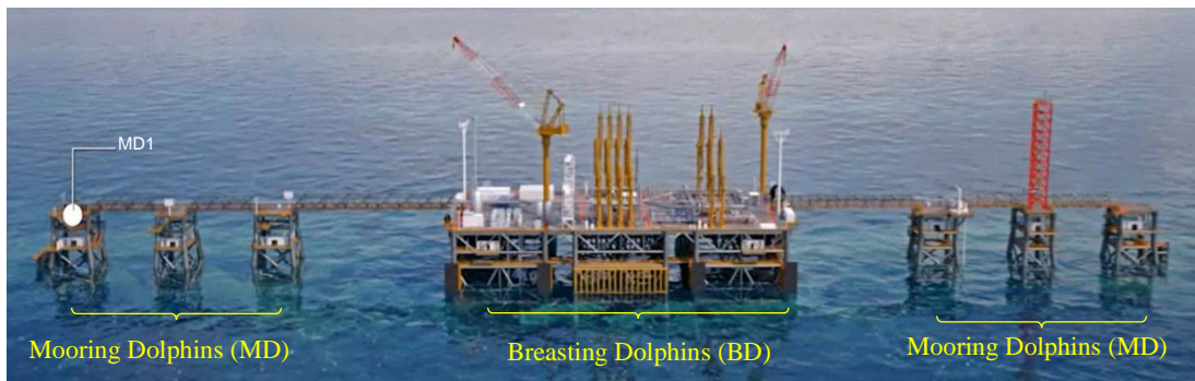
Figure 2: General Arrangement of Jetty
