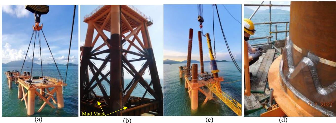
the seabed, and was temporarily supported on the seabed by two large mudmats prefabricated onto the base of the jackets, **Figure 8(a) & (b)**. Once the jacket was lowered to be seabed, it would be difficult to adjust its location or orientation hence for this reason and to ensure safety of the lifting works, the offshore installation required a calm sea state.
