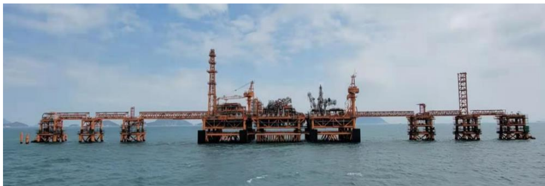
Figure 3: Site Photo of Jetty
