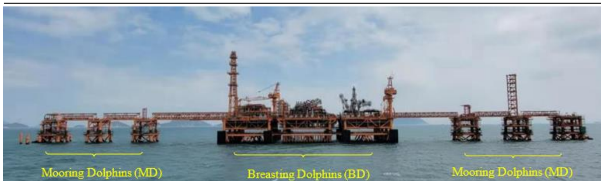
Figure 1: Photograph of the completed foundations of HKOLNGT
