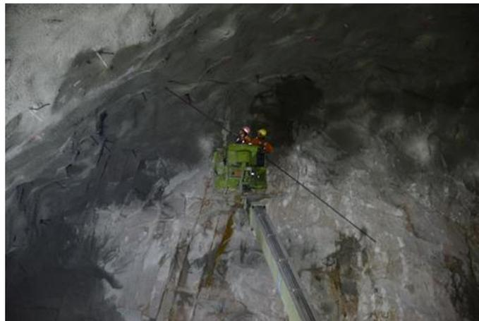
**Figure 5:** Rock bolt installation in hard rock
