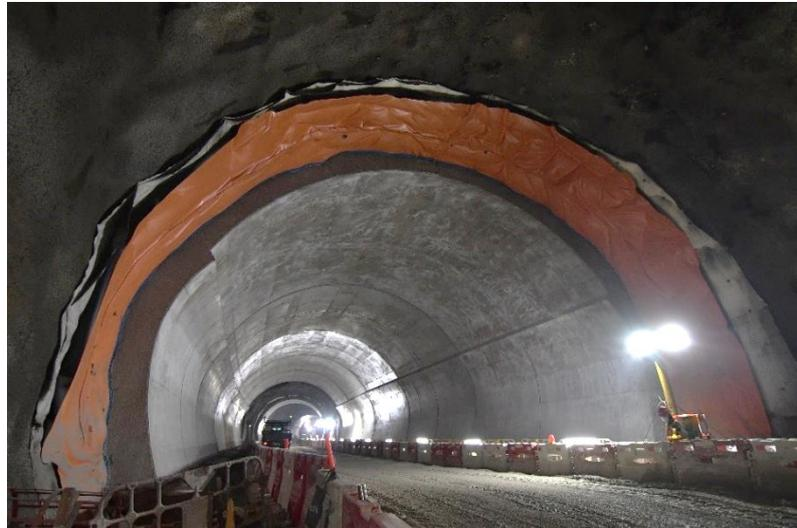
**Figure 4:** Conventional Cast-in-situ Permanent Concrete Lining
