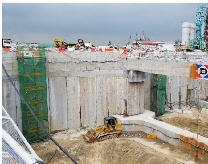
**Plate 1:** Exposed Y-Panel with Struts and Arch Cells
