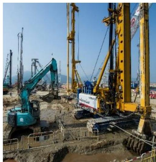
**Plate 2:** Cutter Soil Mixing for Y-Panel
