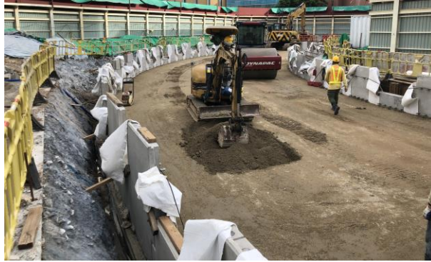
Figure 4d: Placing selected backfill
