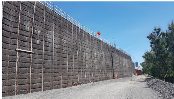
Figure 10: Two-stage construction of Reinforced Earth
