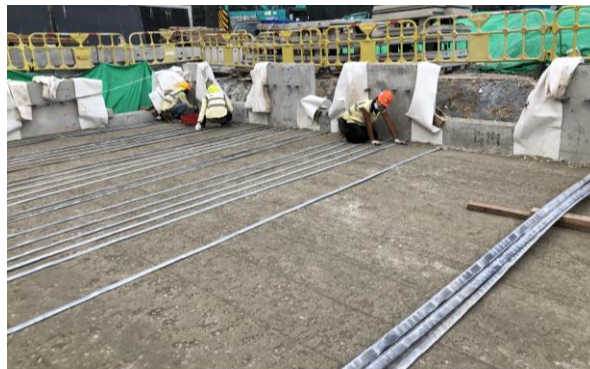
Figure 4e: Placing reinforcing strip
