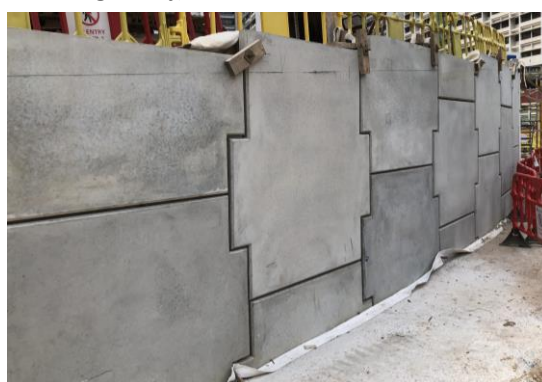
Figure 4h: Completion of Reinforced Earth wall
