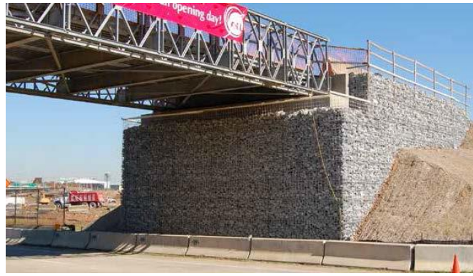
Figure 8: TerraRet Reinforced Earth True Abutment
