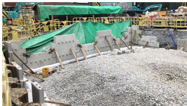
Figure 4c: First layer of panel
