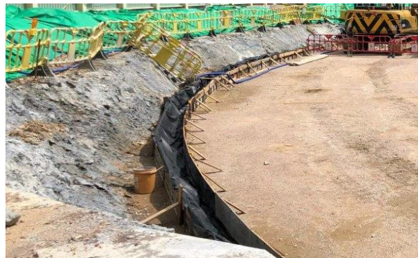
Figure 4b: Leveling Pad
