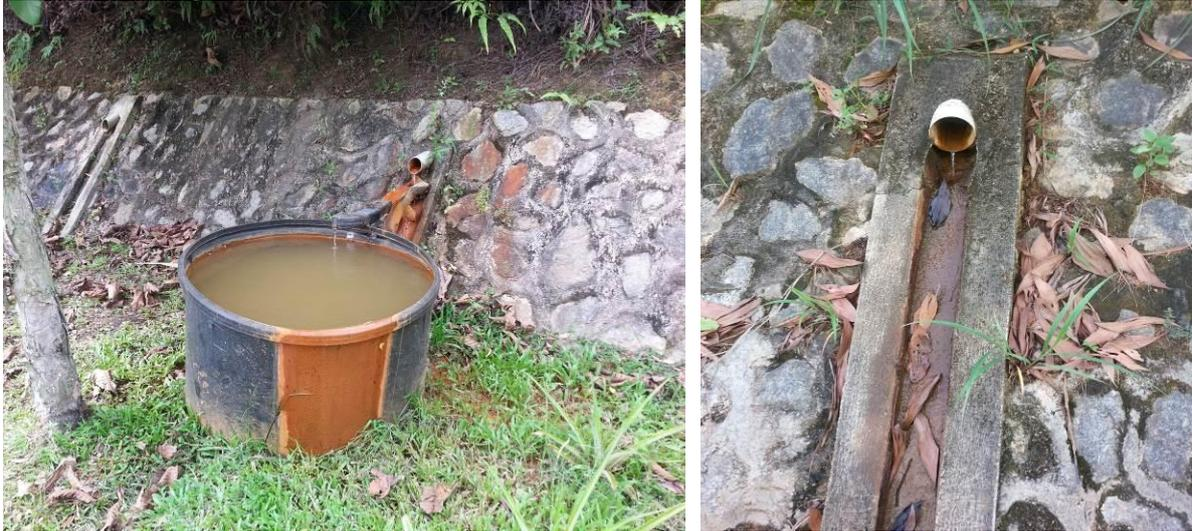
**Plate 1:** Continuous discharge of groundwater from the horizontal drains on site
