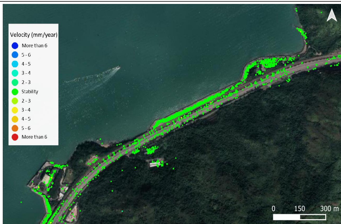
Figure 4: Velocity of deformation map showing stability in a road located at South-West Hong Kong
