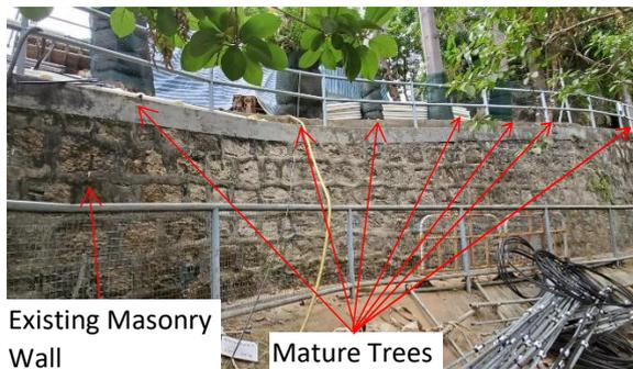
**Plate 1** A tree group at the crest of the masonry wall
