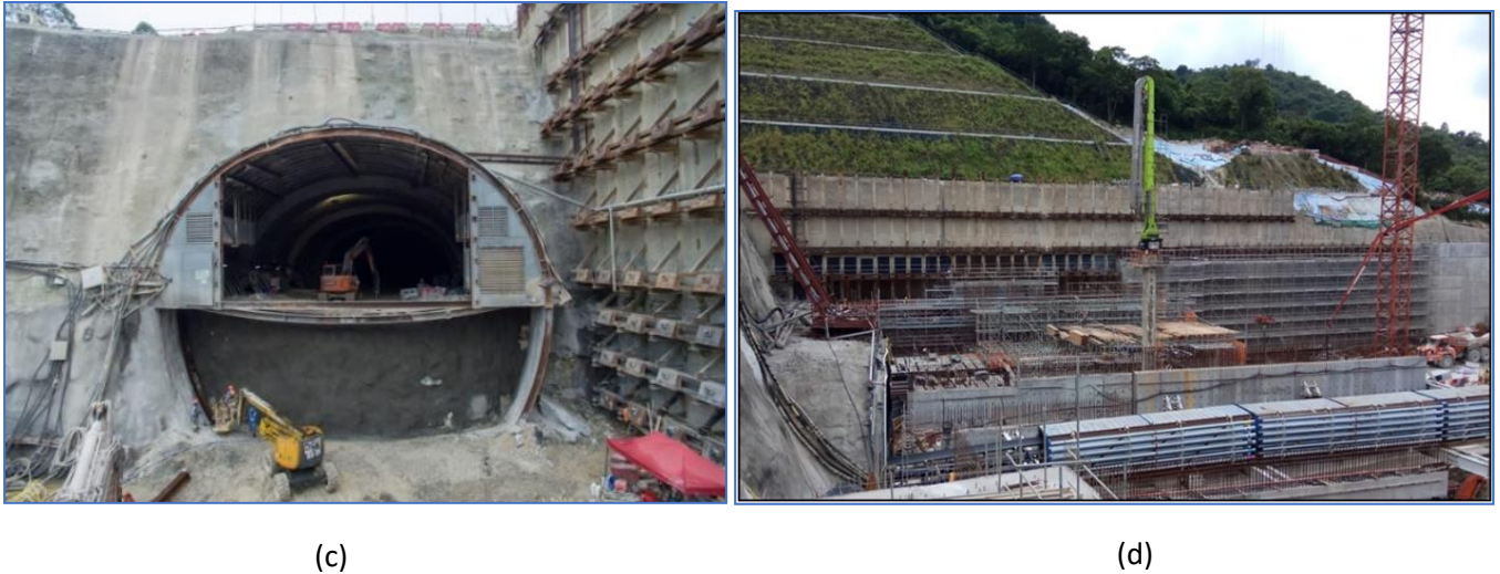
Plate 4: Construction of composite retaining wall at Northern Portal
