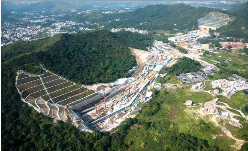
Plate 1: Aerial view of Northern Portal taken in the end of 2016
