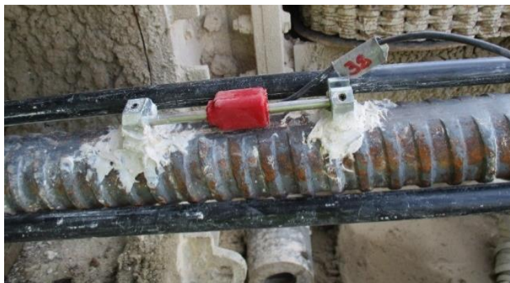
Plate 5: Strain gauge installed on a tie-back
