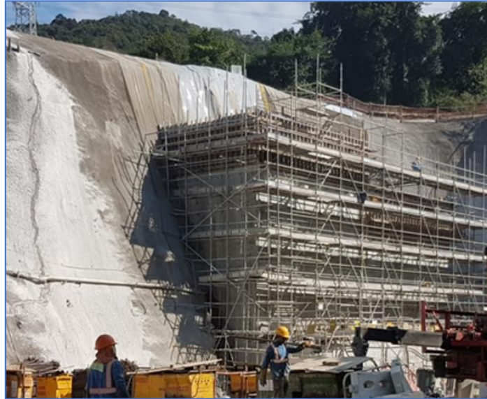
Plate 3: Construction of goose-shaped wall in progress
